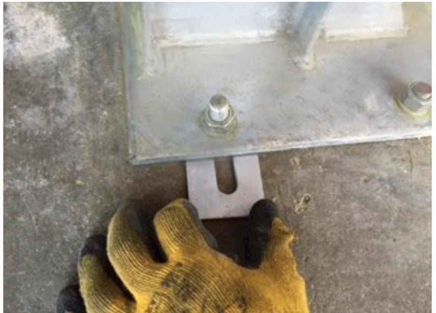
*Trouser Shim being inserted under a base plate to align and level the vertical post.*
