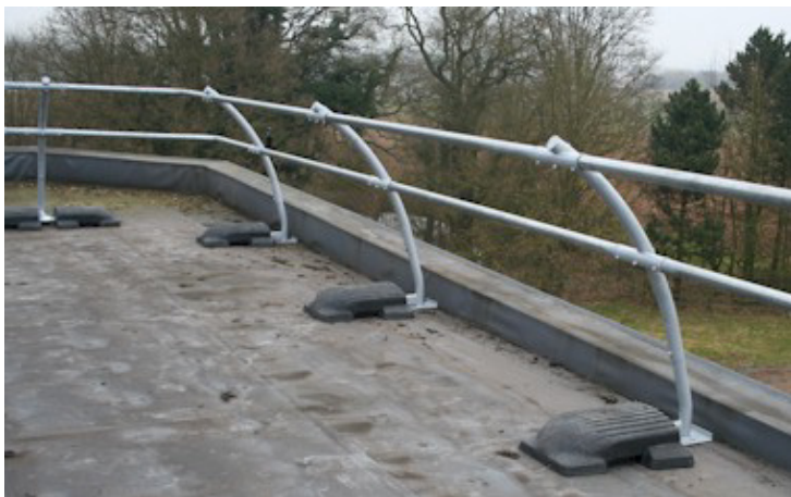
Below Galvanised Steel, with curved posts, 2 rail and 3 rail combinations
