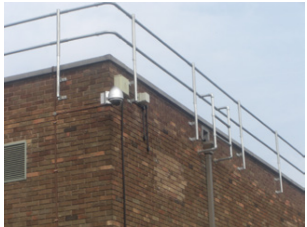
Above Fixed system Galvanised Steel, with bespoke posts affixed to the perimeter of the roof.
